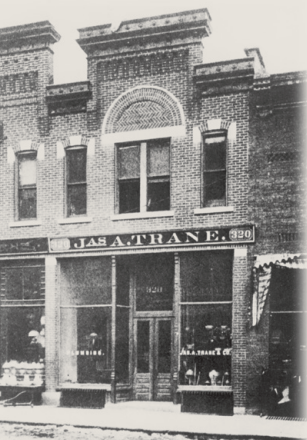
Trane Storefront La Crosse, Wisconsin 1891
